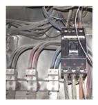
Bad electrical connections due to any loose or corroded terminals, which can generate heat. Measuring this temperature with a safe, noncontact infrared thermometer will help to identify any trouble spots quickly & effectively.
